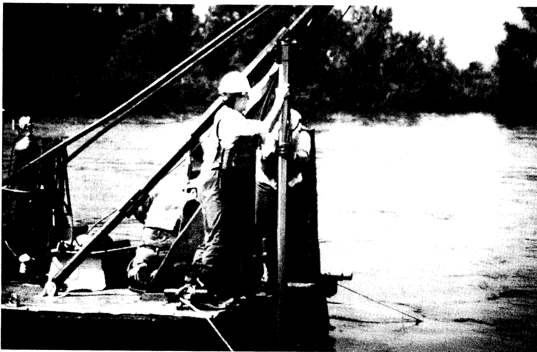
Figure 4. A-frame used during vibracore process
