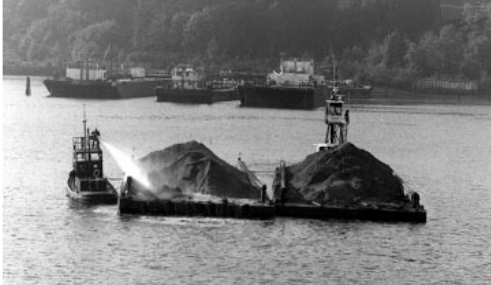
Figure 5. Pressure-hose washing method of placement
