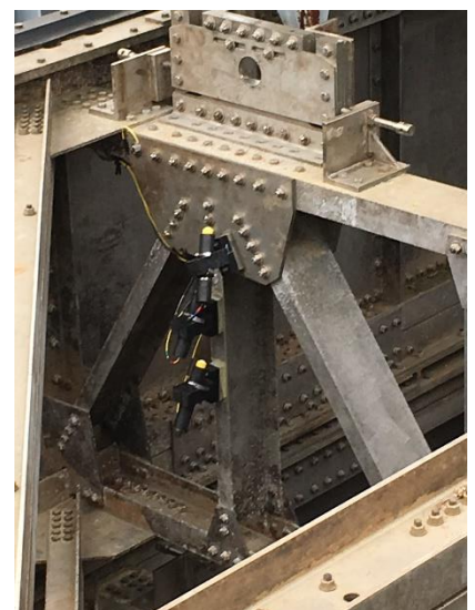
Corrosion sensors mounted on emergency bulkheads
