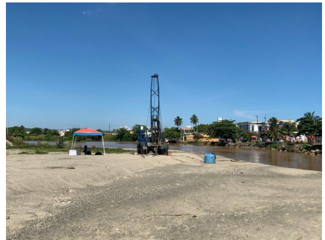
Figure 1: Example of Project Boring Site
