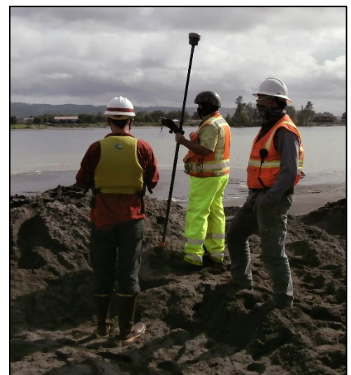
Figure 2. Examples of standard safety gear for Quality Assurance Representatives working on a dredging job.
