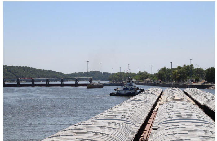
Figure 2. Upstream approach to existing 600-ft long chamber
