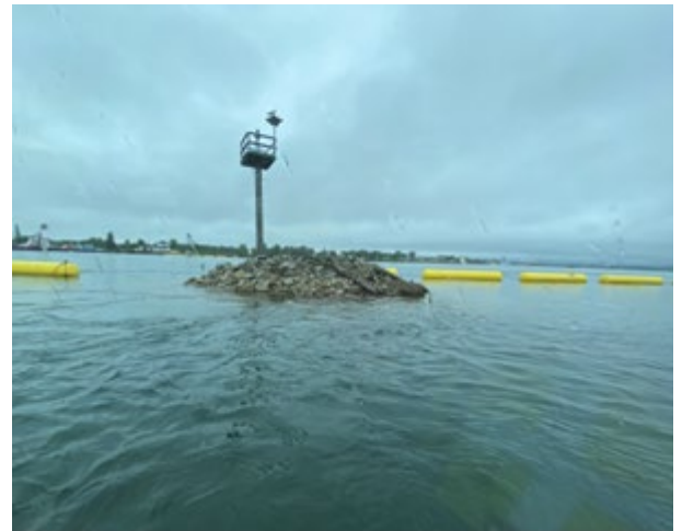
Figure 1. Ice island with displaced H-pile anchor. Ice booms in the background.
