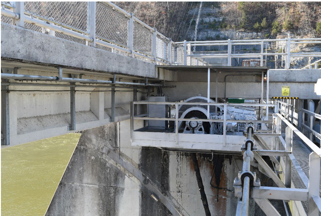
Figure 1. Existing mechanical platform at the Cordell Hull Dam.
