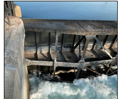
Figure 1. Two dead lake sturgeon trapped on the lower girder of the compensatory gate closest to the bank at the St. Marys River Project.
