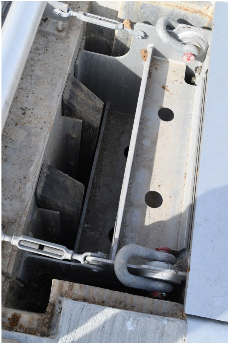
Figure 7. Depth locating angle iron on existing protection plate.
