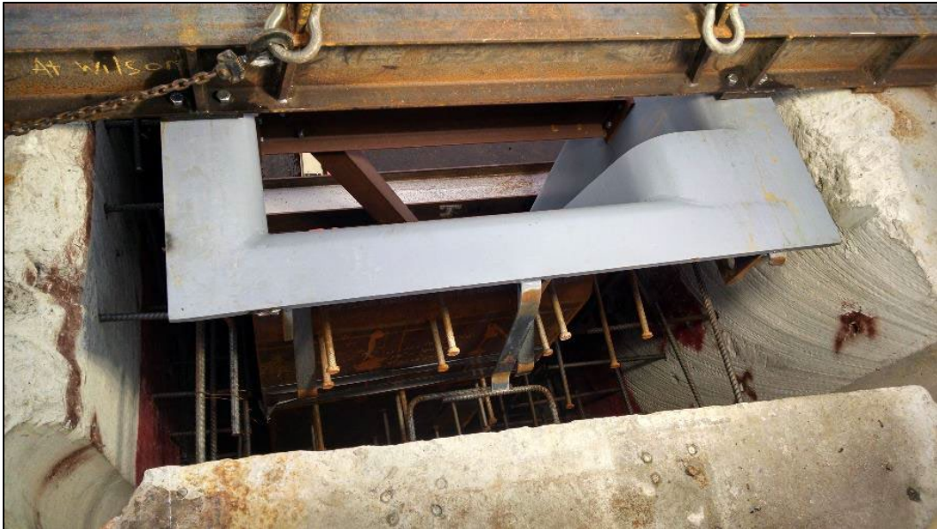
Figure 5. Installation of 110-ft. slot armor prior to concrete pour.
