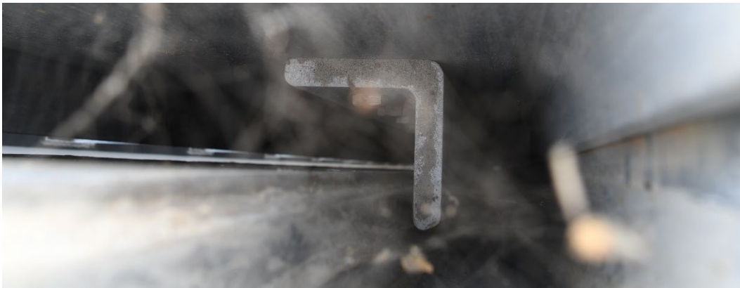
Figure 7. Depth locating angle iron on existing protection plate.
