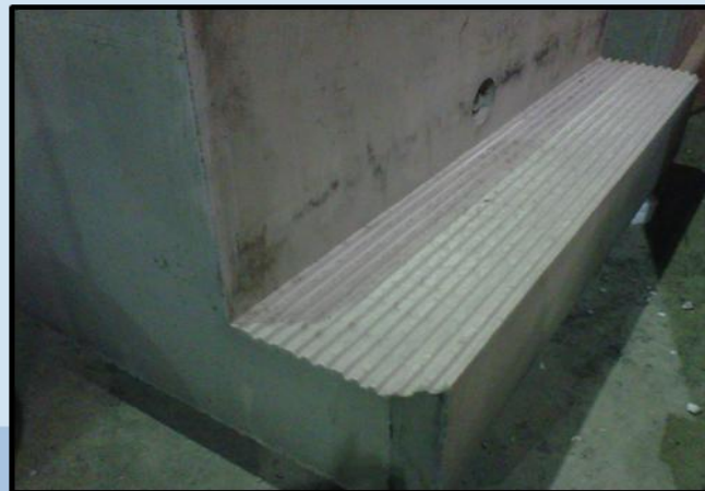
Environmentally Enhanced Breakwater Toe Blocks
